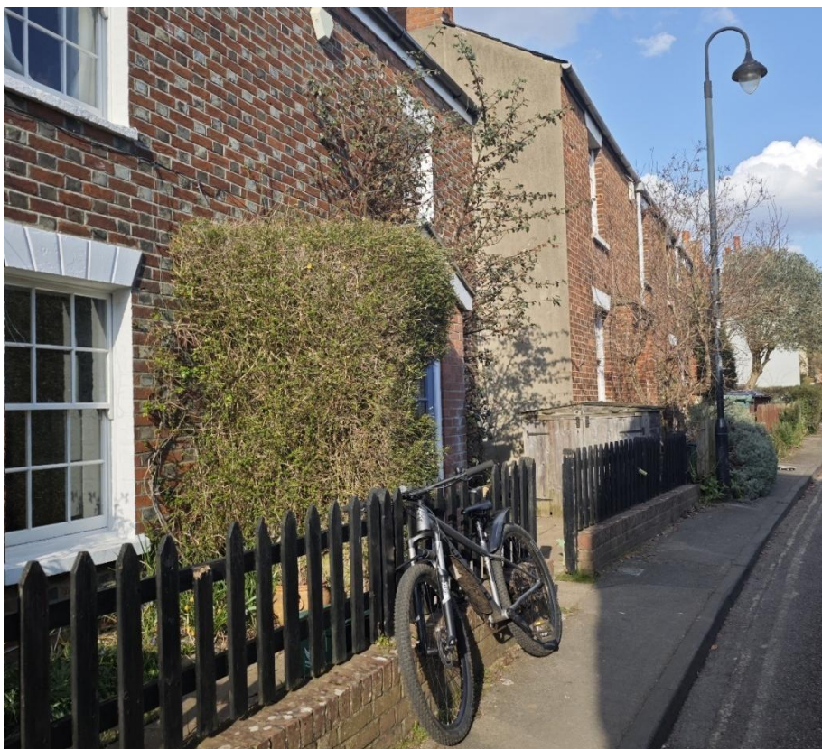
Figure 21: Low Brick Walls topped with palisade timber fencing are common within the conservation area
