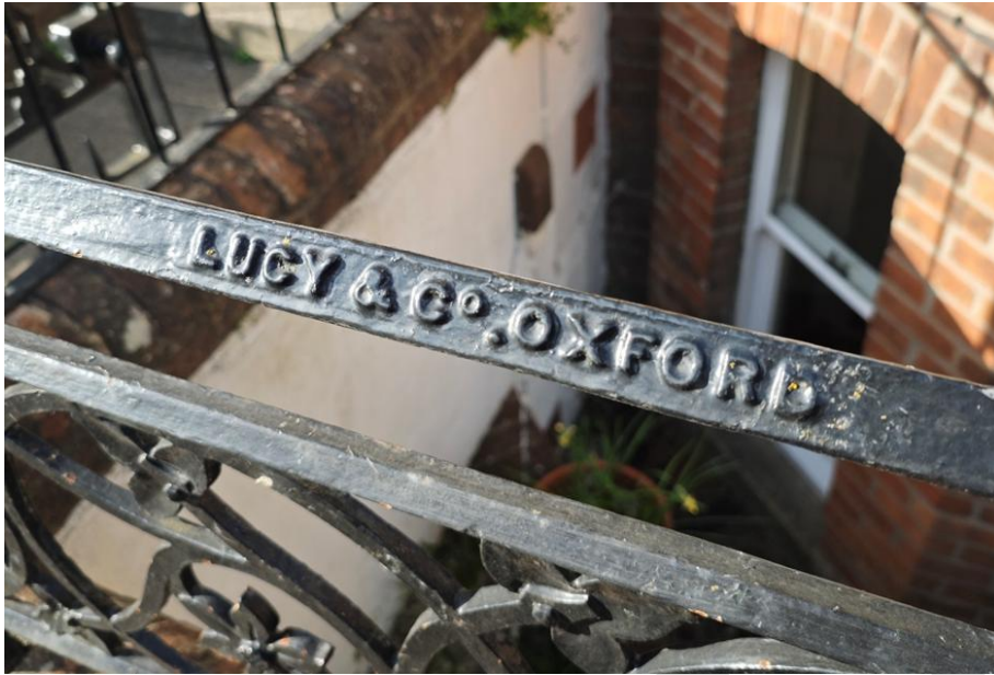
Figure 23: Traditional Iron Lucy and Co. Railings at 4-8 St Bernard's Road.
