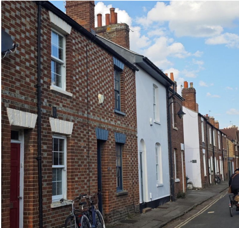
Figure 87: Roof alterations can disrupt uniformity and erode detailing at eaves and ridge height if not addressed sensitively
