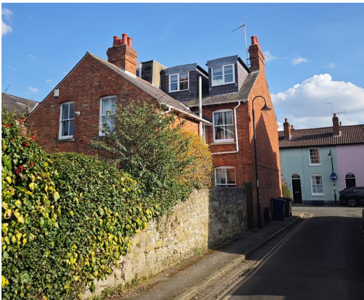
Figure 44: Greenery to rear gardens which is visible from Adelaide Street softens the otherwise hard streetscape. Instances of stone boundary walls also add texture to character area
