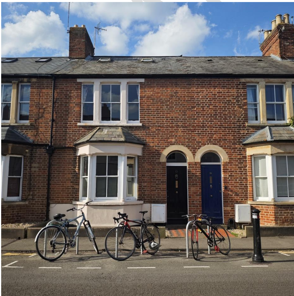
Figure 81: New cycle parking on Observatory Street
