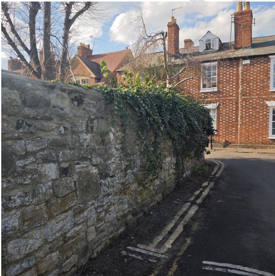
Figure 24: Individual instances of stone walls are found within WMCA. Pictured: Rear boundary stone wall on Adelaide Street
