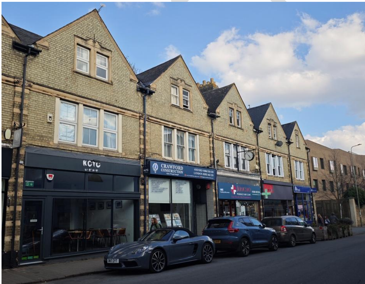
Figure 65: Shopfronts at 112-118 Walton Street have been replaced unsympathetically, losing their uniformity and cohesion and ultimately detracting from their appearance.
