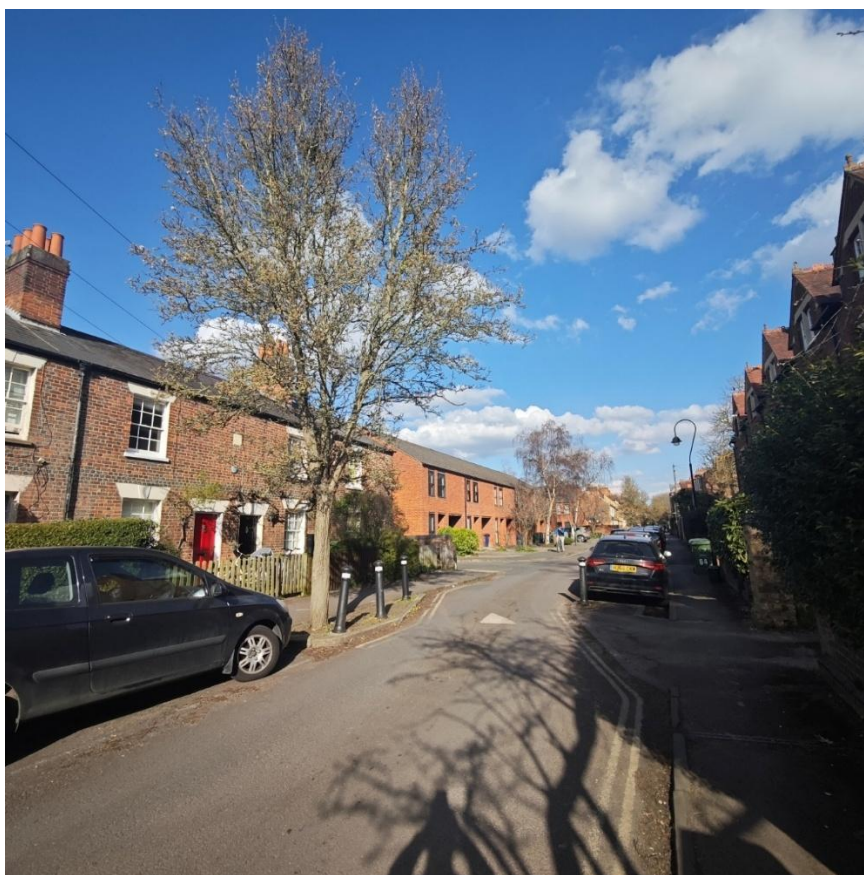
Figure 14: Ornamental Greenery and individual instances of trees within the public realm soften the streetscape. Pictured: St Bernard's Road
