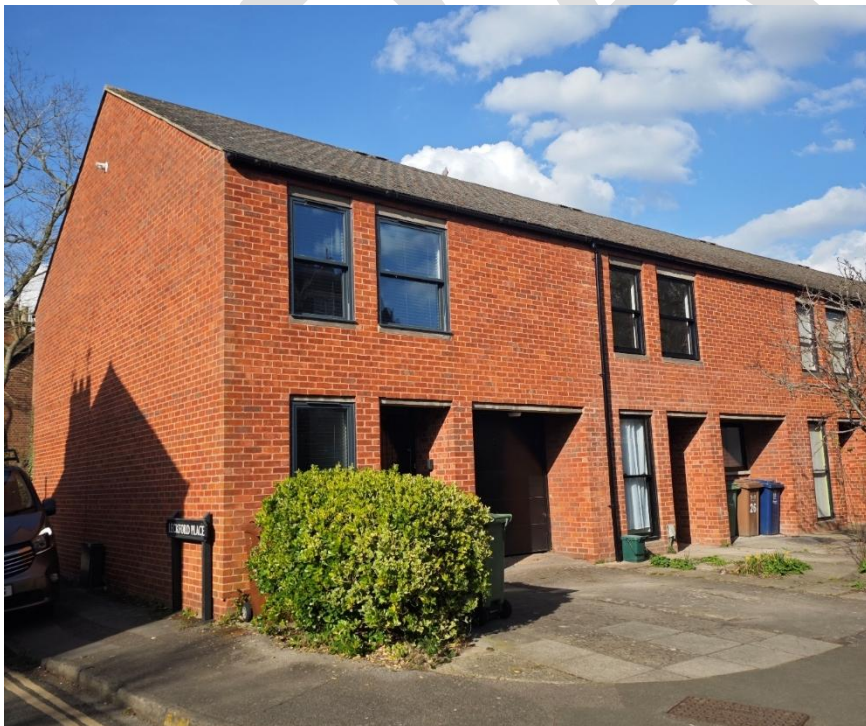
Figure 26: More modern terraced blocks imitate scale, material and uniform pattern of fenestration. Pictured: Terrace dwellings at Arthur Garrard Close, St Bernard's Road
