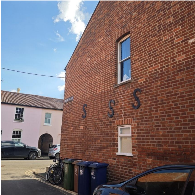
Figure 17: "S" shaped pattress plates at corner of Observatory Street and Adelaide Street
