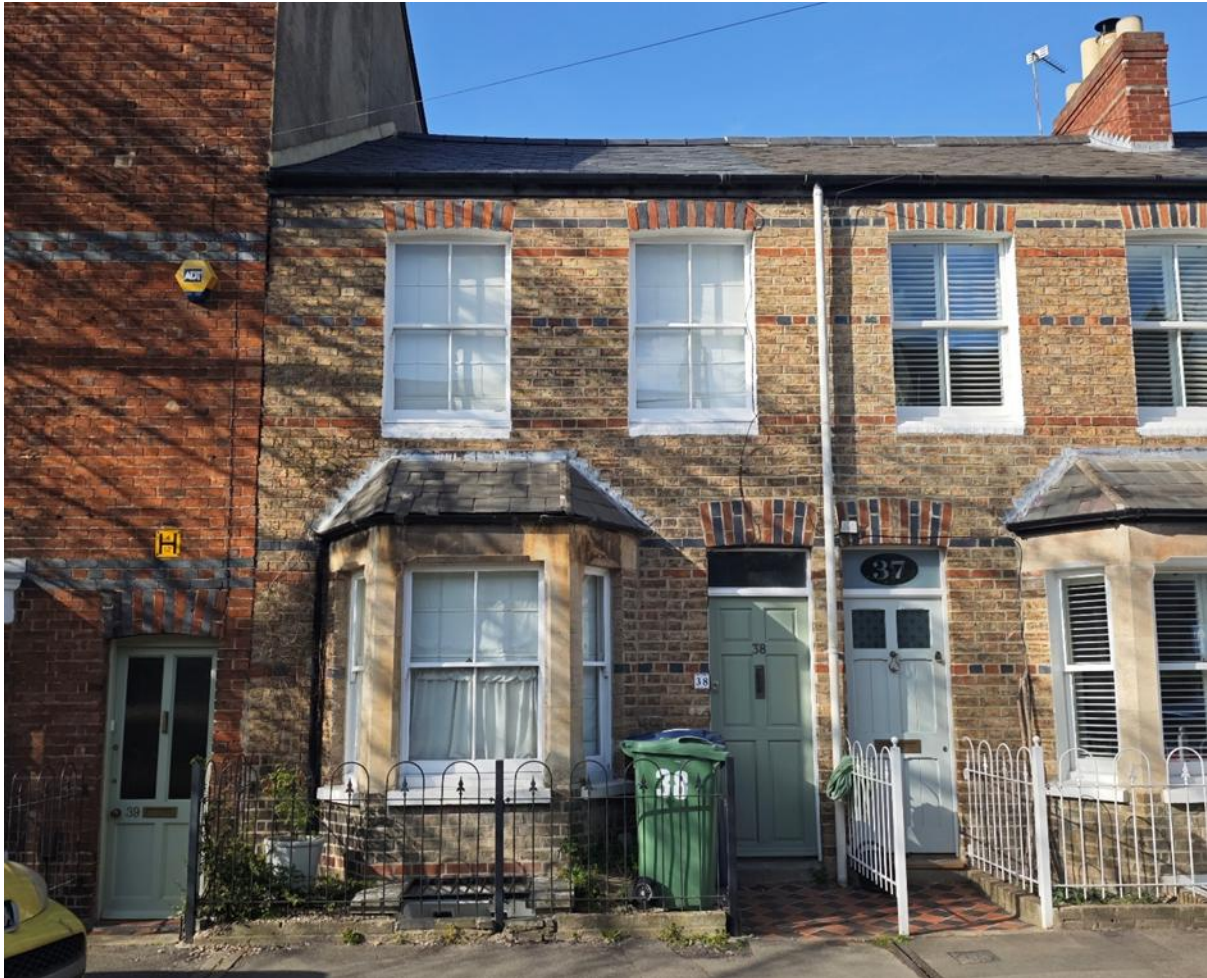
Figure 37: Bay windows become more prevalent further north in the Conservation Area. Decorative brickwork is evident and 2-over-2 windows are more common. Pictured: 38 St Bernard's Road
