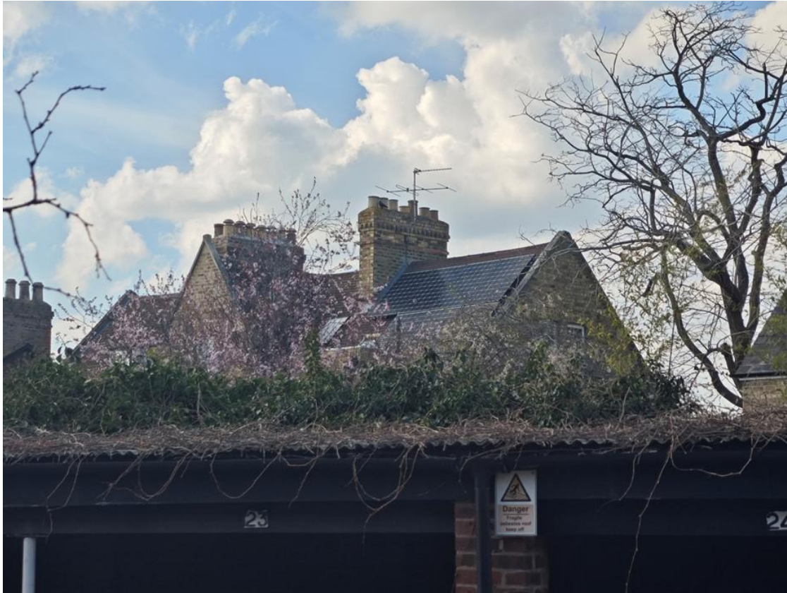
Figure 83: PV Panels to rear roofslope of 60 St Bernard's Road- only visible from resident's garage at Walton Manor Court
