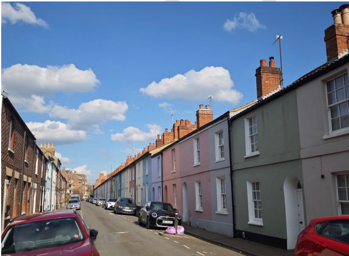
Figure 35: Observatory Street: Georgian Terraces: repetitive fenestration, painted panelled front doors with fanlights and traditional sash windows
