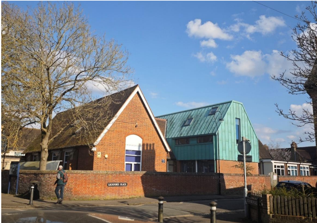
Figure 31: Leckford Place School on corner of Leckford Place and Leckford Road
