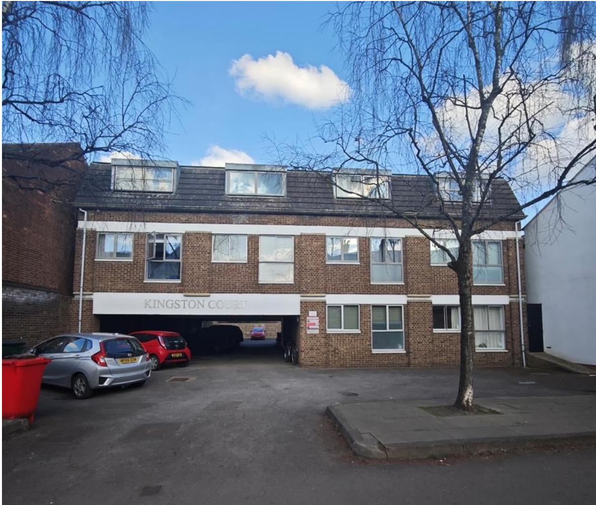
Figure 66: Kingston Court, a 1970s block of flats is set back from pavement, disrupting street pattern.
