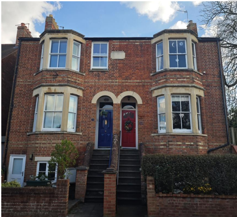
Figure 28: Grander Semi-detached dwellings with basement space at 73-74 St Bernard's Road
