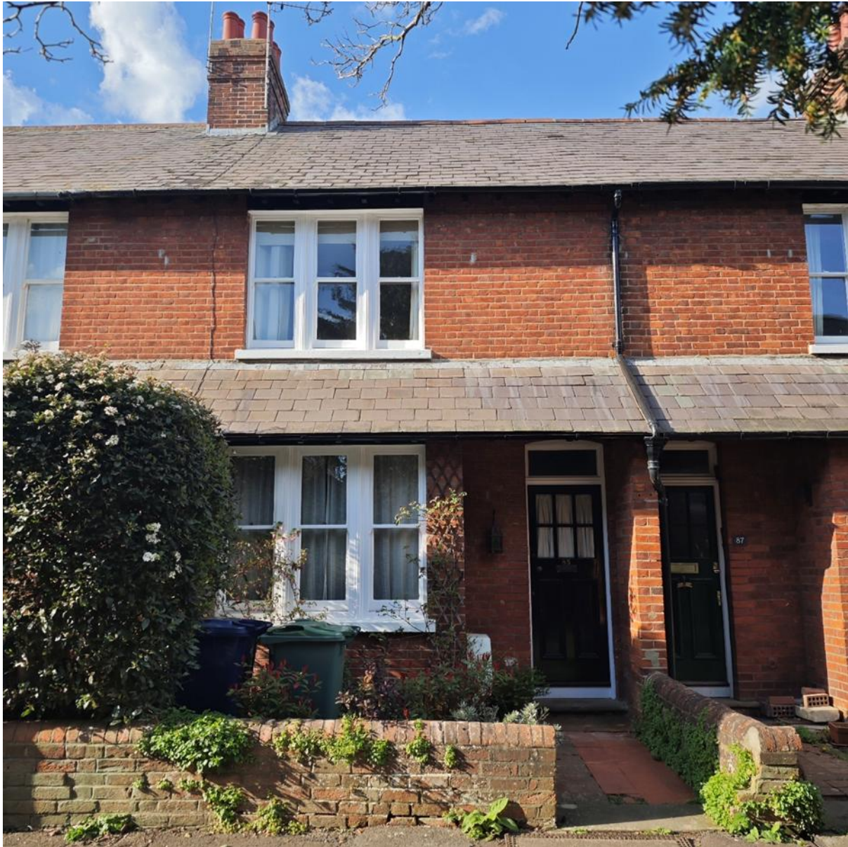
Figure 51: Low brick boundary walls are common throughout the area
