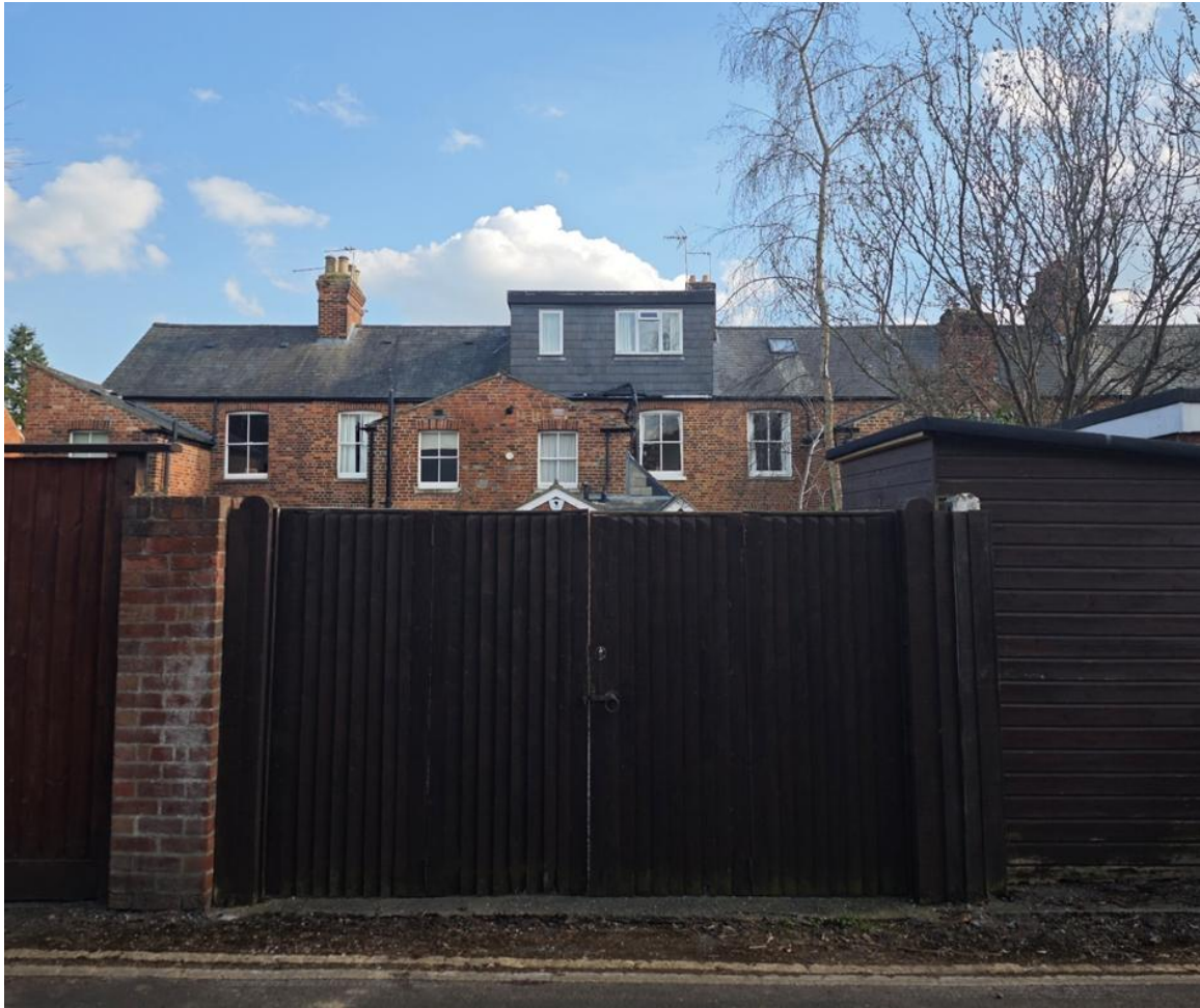
Figure 70: Overly large dormers to rear roofscapes with unsympathetic flat roofs can appear as a third storey instead of a "room in the roof".
