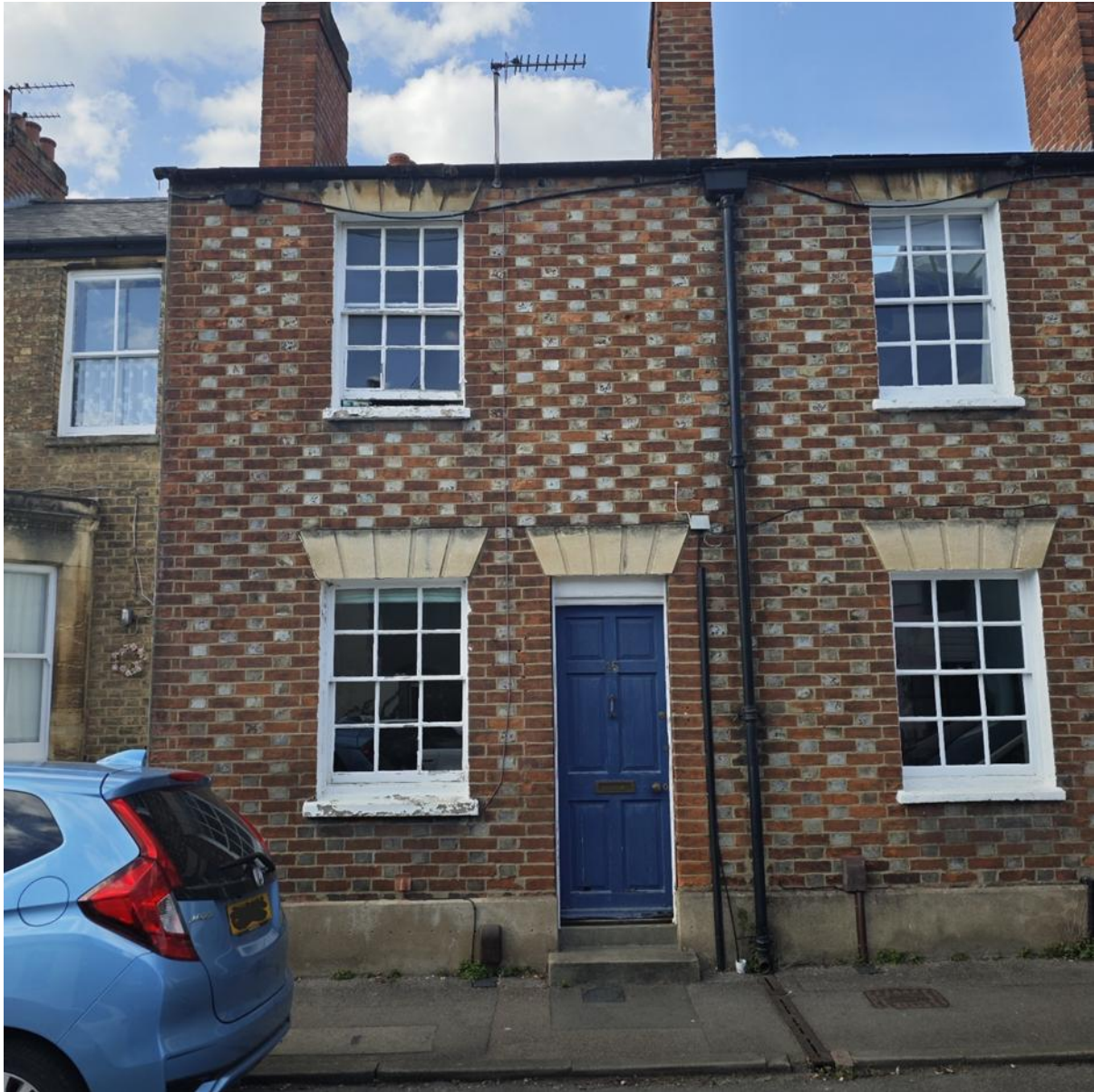
Figure 36: Terraced workers cottage on Observatory Street: diaper brickwork, decorated stone lintels above windows and doors, traditional 6-over-6 sash windows
