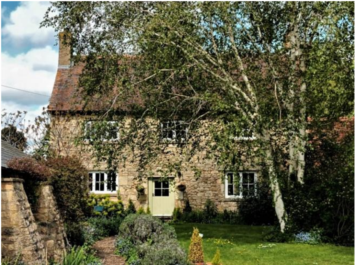
Figure 44: Manor Farmhouse (Perch Cottage)
