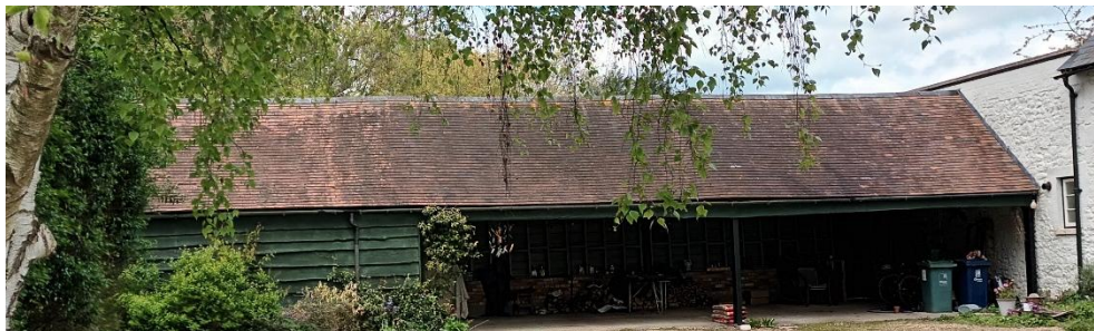
Figure 37: Red clay tiles on outbuilding roof at Manor Farm
