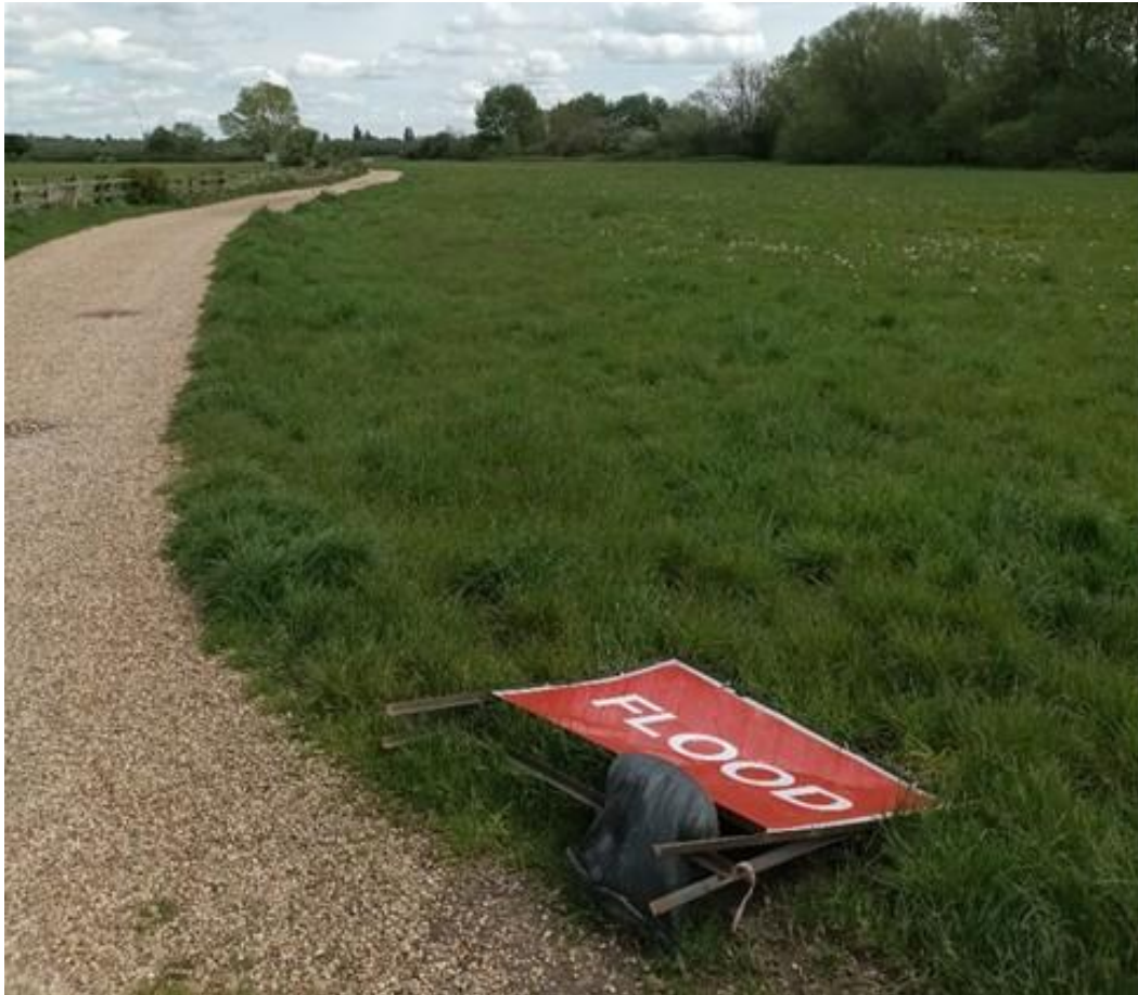
Figure 41: Flood warning sign on the pubic path along Binsey Green
