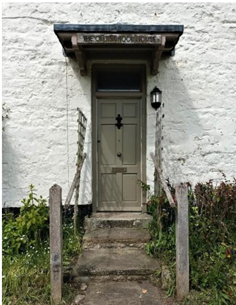
Figure 34: Six panelled timber door, The Old School House
