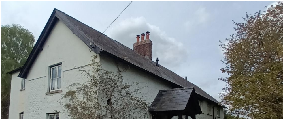
Figure 36: Welsh slate roof and tall brick stack at Manor Farm
