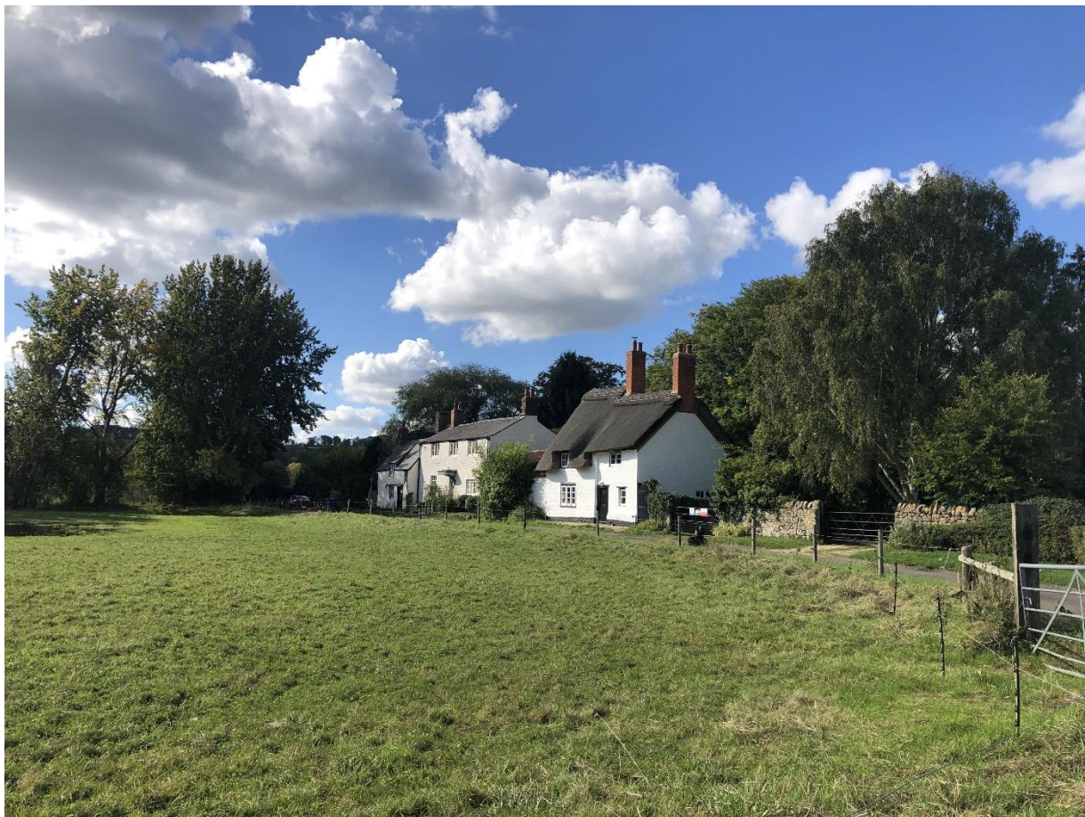
Figure 2: View of Binsey Cottages
