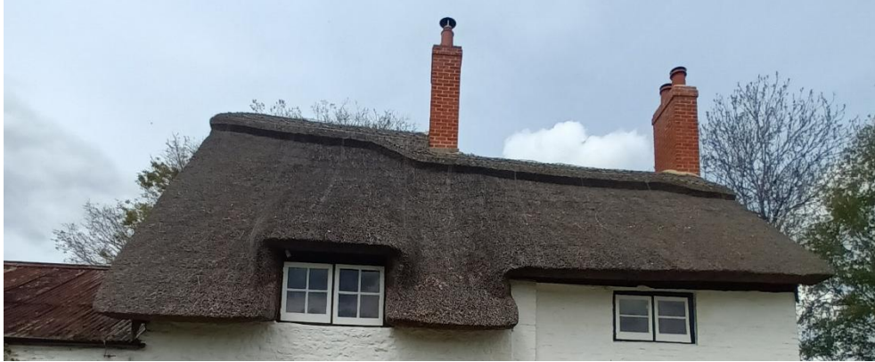
Figure 35: Thatched roof and tall brick stacks at The Thatched Cottage.
