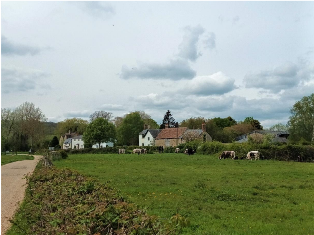
Figure 20: View of the row of buildings as seen from the pedestrian path along Binsey Green.
