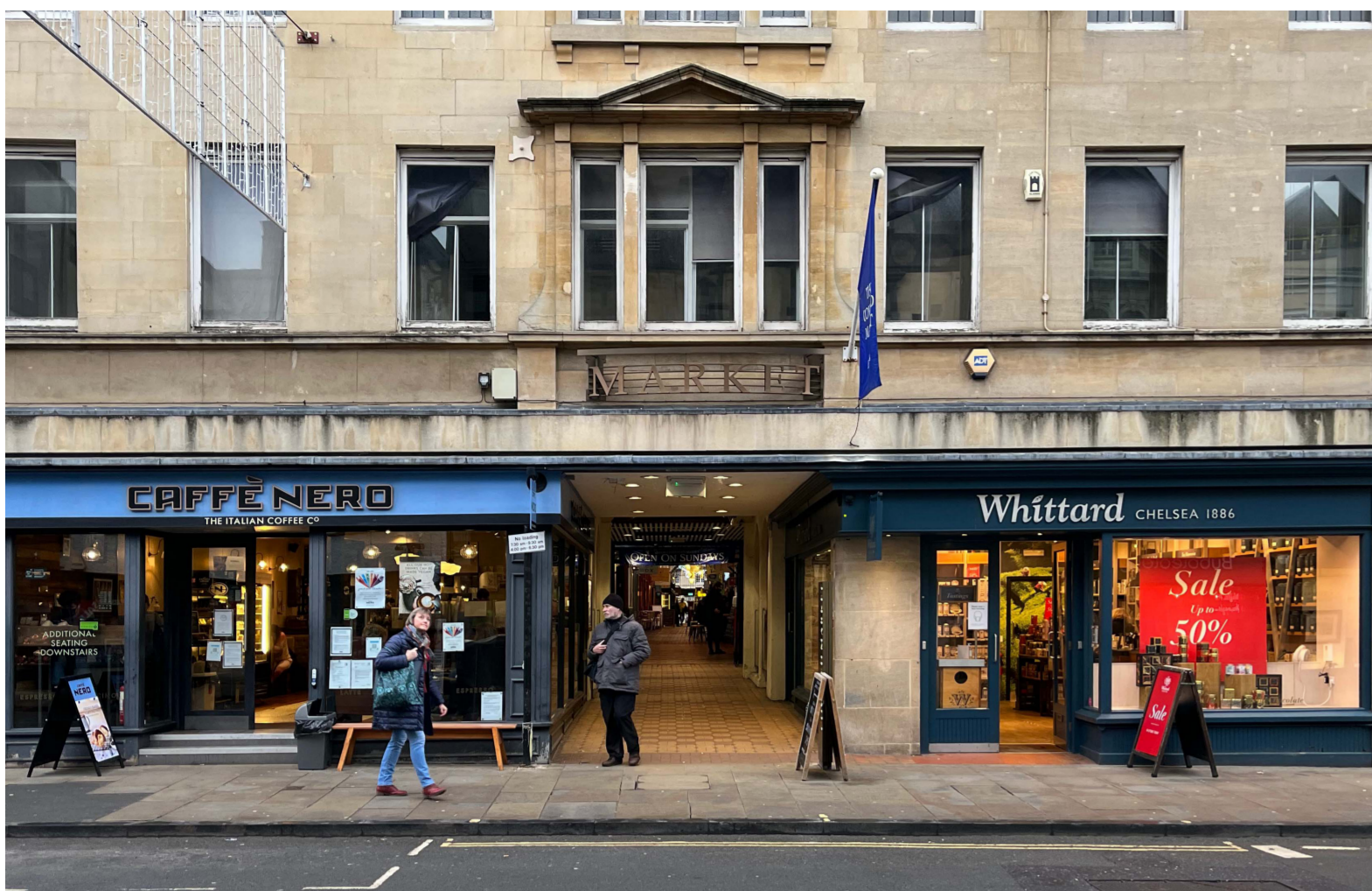
Existing view of one of the entrances from the High Street
