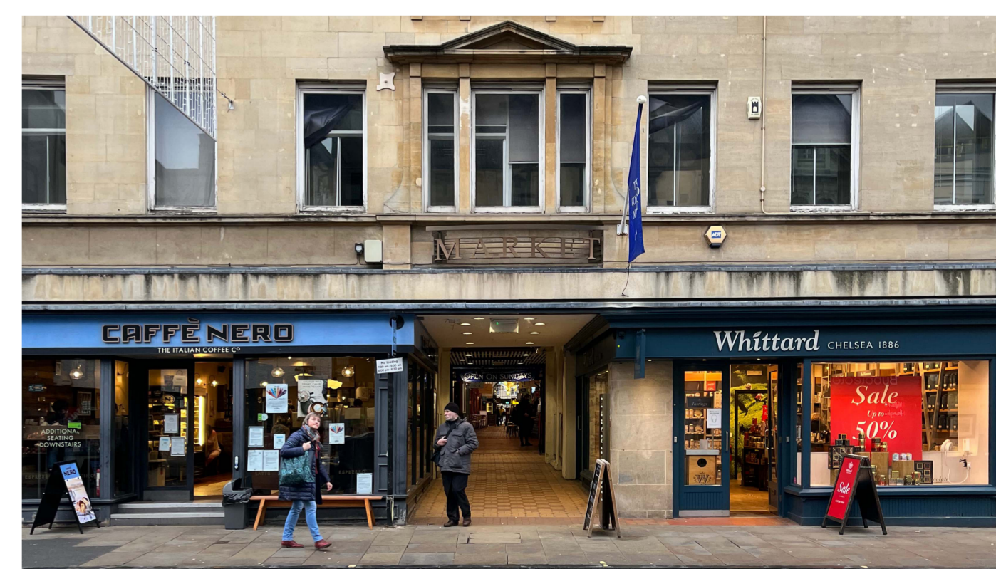
6. High Street entrances: Cluttered with poor visibility/signage
