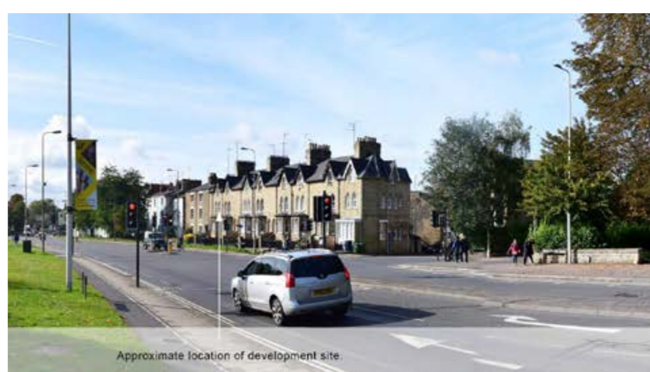
Existing View from Headington Road
