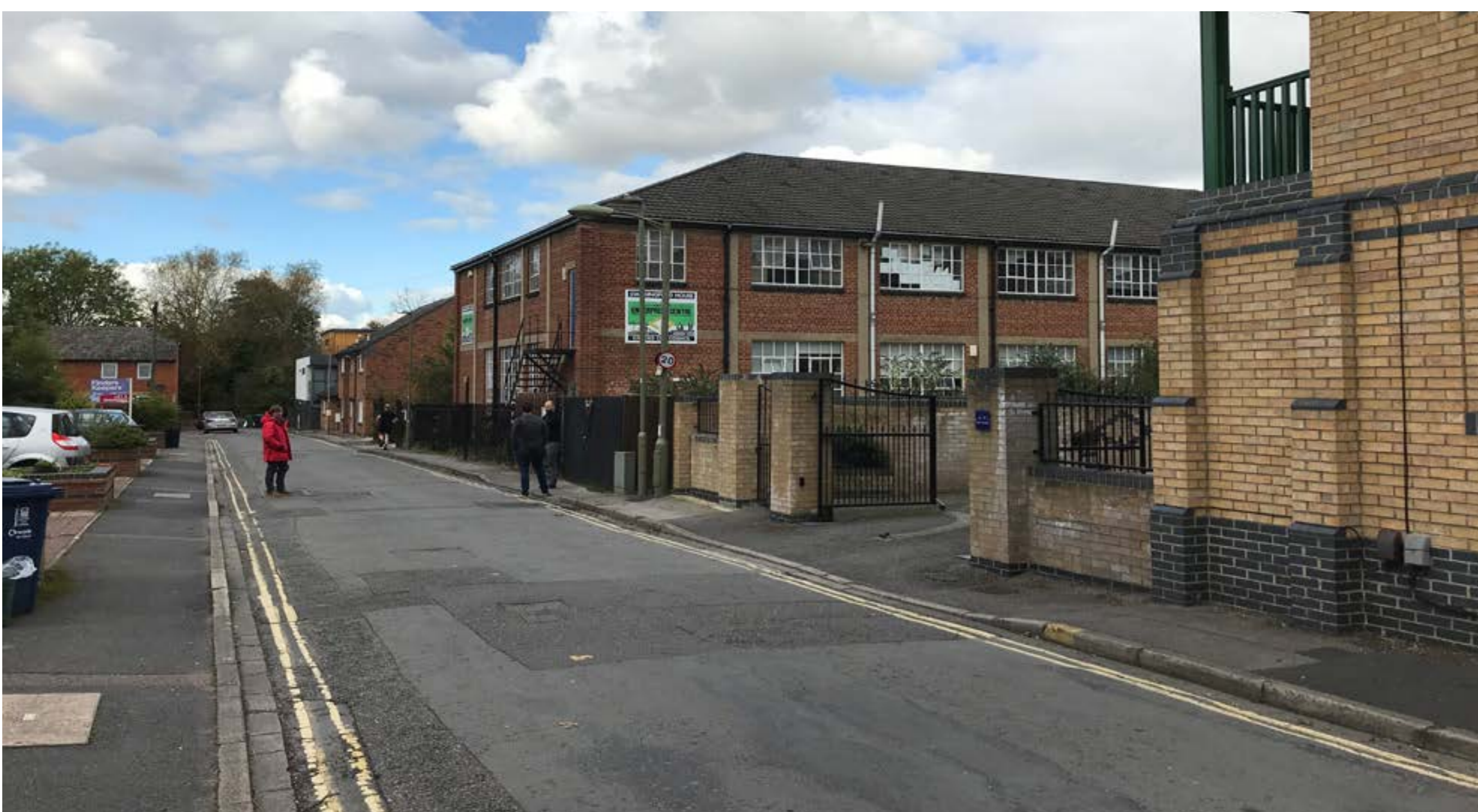
View of the existing building from Cave Street
