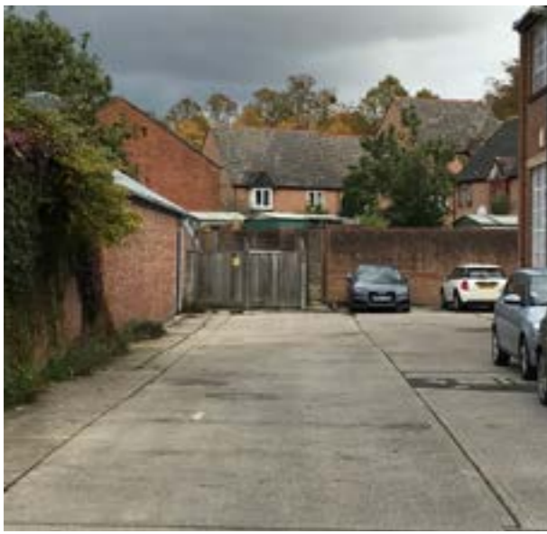
Existing site materiality
