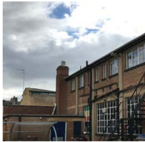
Existing site materiality
