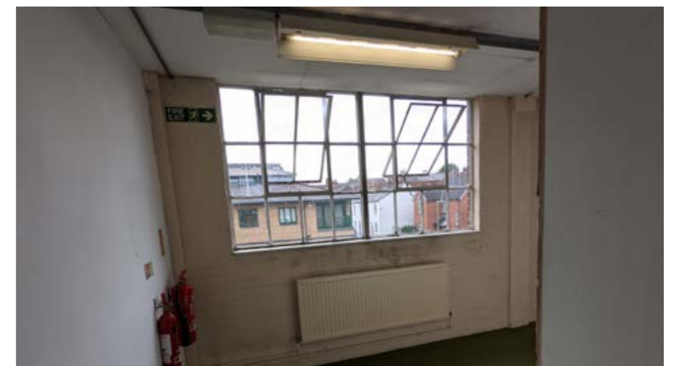
Internal view as existing
