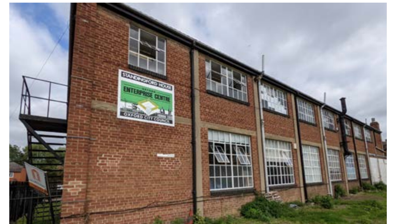
External view as existing
