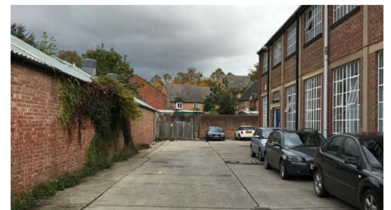
External view of the building as existing
